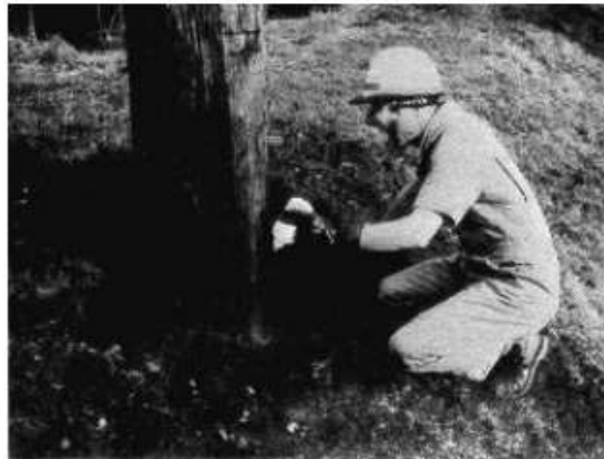
Figure A-1. Applying Vapam treatment.
